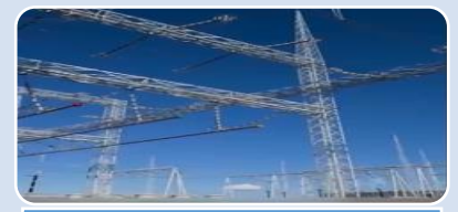
An innovative solution to solve the electricity imbalance
